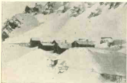
Jumbo Camp, the scene of the disaster which wiped out half the buildings of the mine, killing several men and injuring many more. The barricade, or "snow divider" at the extreme right was supposed to sidetrack avalanches but in this case the snow poured right over the barricade. K7BLLI was located in the long building at the right.
